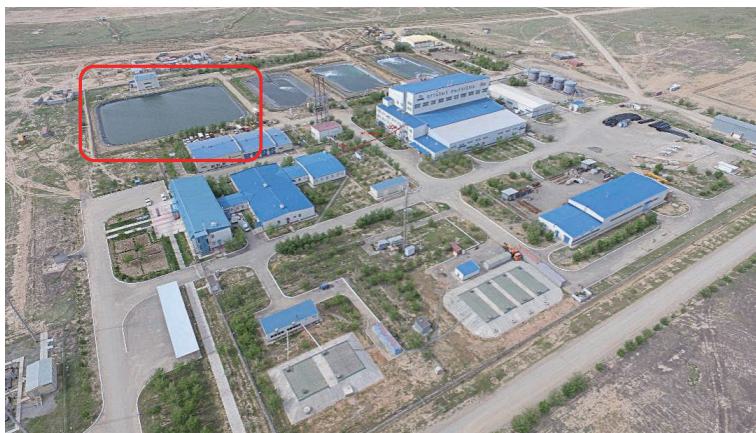
Note: Domestic wastewater treatment (red circle) 附註：生活廢水處理(紅框)
